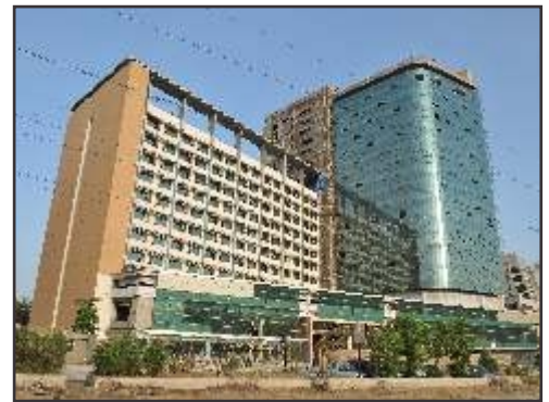
Shapath V Tower, Ahmedabad
